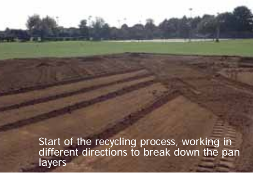
Recycling the original loam and grading of the new pitches
