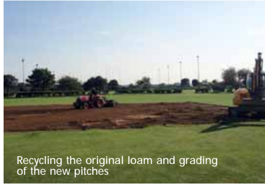
Cultivated soil just prior to rebuilding the square with the laser grader
